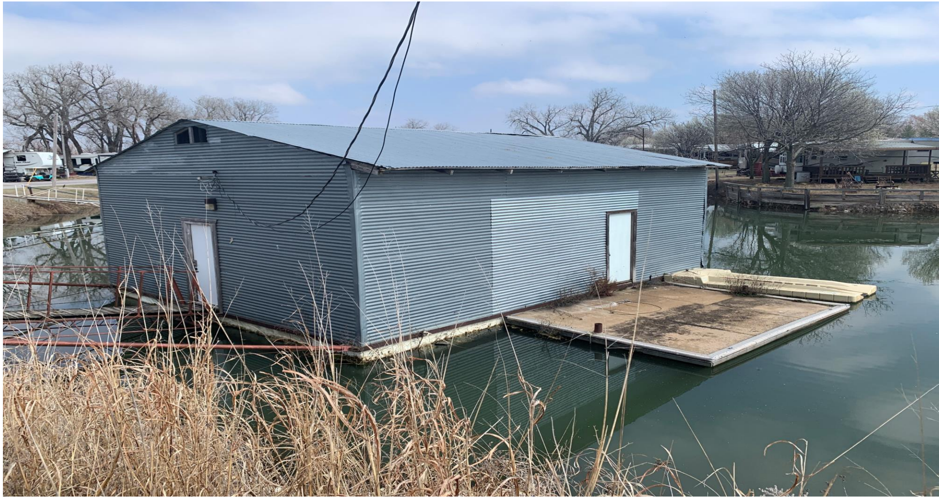
Wet Slip photo 1
